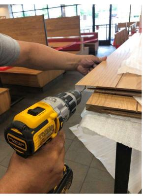
5. Slide panel down over the alignment flanges/splines of the posts.
