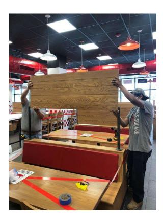
6. Use one rounded-head (shorter) screw, per side, to secure the wood panel to the posts.
